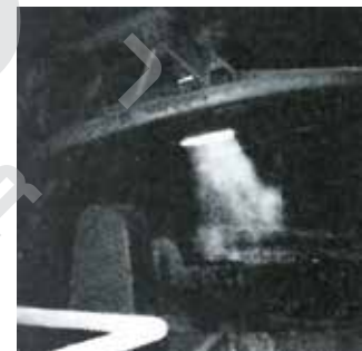
Z-Blok® modules dramatically improved the efficiency of this ladle heat shield, reduced maintenance.
